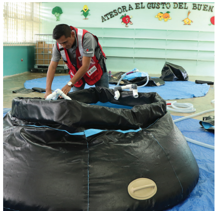
Red Cross worker Jenner Alarcón helps set up and fill an “onion” water storage tank at a local school. The Red Cross provided 43 of these 30,000-liter water tanks to schools in Puerto Rico to provide clean water during emergencies. Photo by American Red Cross
