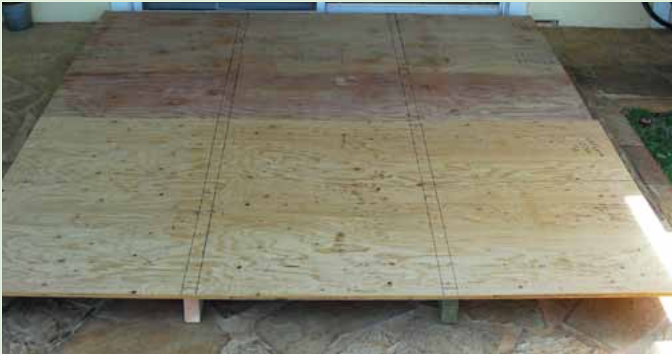
Figure 4-35. During assembly of the shutters in Figure 4-28, the two panels to be joined sit atop the 2 by 4's. The outline of the 2 by 4's and all screw locations are marked on the panel. Panels should be cut, labeled, and marked as to all fastening locations before hurricane season. The panels can be quickly attached with wood screws drilled from the plywood panel into the 2 by 4. The panel is then raised with the end near the window being the pivot point. The panel is then attached to the structural framing of the window as shown in Figure 4-34.
