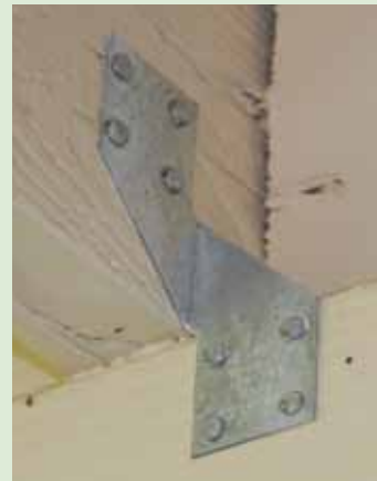
Figure 4-4. This is an example of retrofitting an existing house, originally built without hurricane clips. The popular H3 clip is used here; four nails attach the clip to the roof (truss-rafter) and four more nails attach to the wall or top plate below. For a retrofit, the clips are exposed on the outside of the house, therefore, both the clip and fasteners should be corrosion resistant and painted to blend with the exterior of the house. With the correct clip and nails you could perform the work or, if you prefer, hire a licensed contractor. 23
