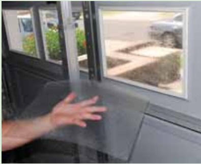
Figure 4-22. Laminated film comes in various thicknesses and strengths. Here the film is applied to an existing window before it is fastened to the frame with silicone structural sealant.
